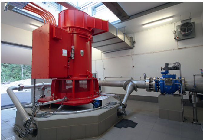
Icogne (CH) 4-nozzle turbine, used in an irrigation system ( Q = 0.473 \text{ m}^3/\text{s} , H_n = 479 \text{ m} , D_{ext} = 1018 \text{ mm} , 1000 \text{ rpm} , P_m = 1996 \text{ kW} )
