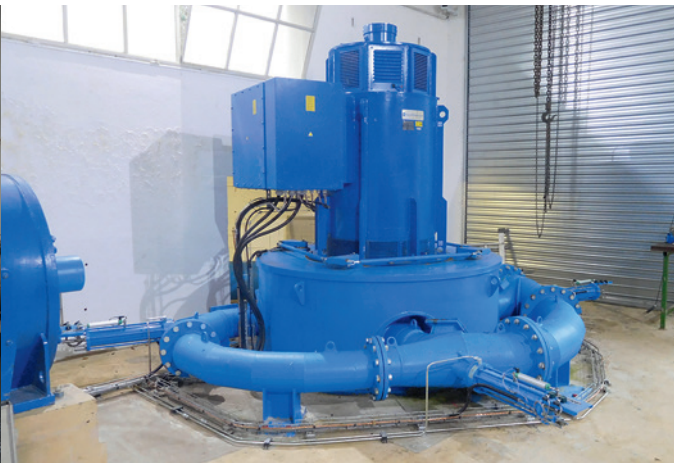
Lafarge (France) 4-nozzle turbine set up with a manifold in the runner's plane ( Q = 0.590 \text{ m}^3/\text{s} , H_n = 85 \text{ m} , D_{ext} = 838 \text{ mm} , 600 \text{ rpm} , P_m = 435 \text{ kW} )
