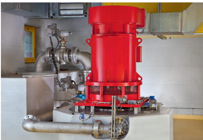
Profray, 2-nozzle turbine, running on raw wastewater ( Q = 0.100 \text{ m}^3/\text{s} , H_n = 430 \text{ m} , D_{ext} = 648 \text{ mm} , 1500 \text{ rpm} , P_m = 380 \text{ kW} )
