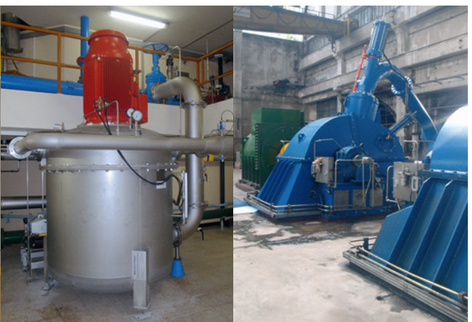
Haute-Pierre (CH) back-pressure turbine, integrated in a drinking- water network ( Q = 0.083 \text{ m}^3/\text{s} , H_n = 104 \text{ m} , D_{ext} = 654 \text{ mm} , 765 \text{ rpm} , P_m = 76 \text{ kW} )
